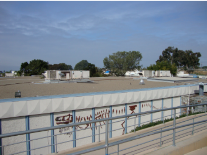
Ramps from Industrial Arts leading to Building 100's
