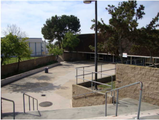
Courtyard Outside of Gymnasium East Entrance
