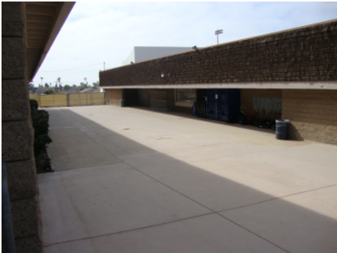
Open Area Between Gymnasium and Locker Room Bldg.
