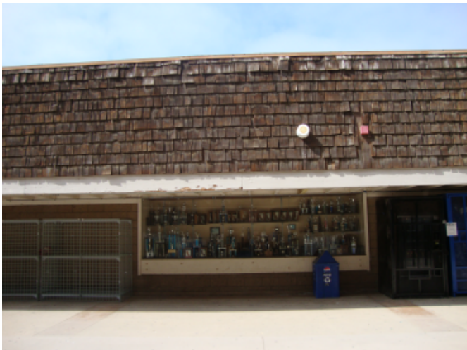
Locker Room Building's East Elevation
