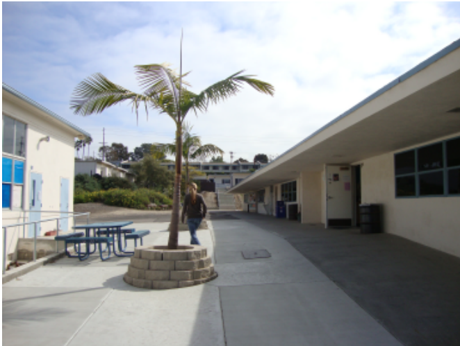
Building 20's on the right, Building 50's on the left
