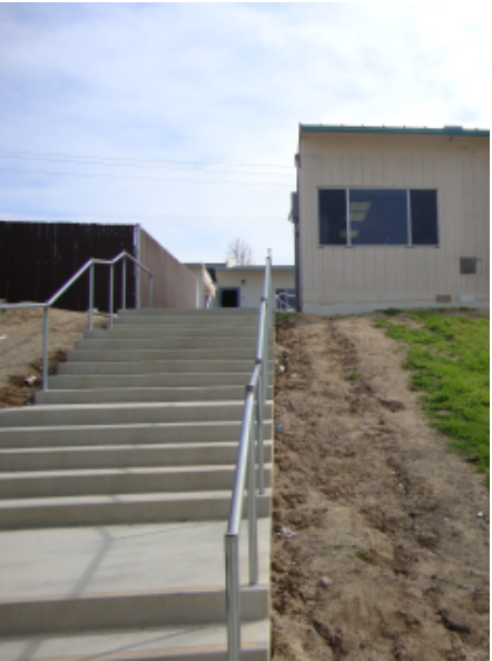
Stairs Leading to Building 30's
