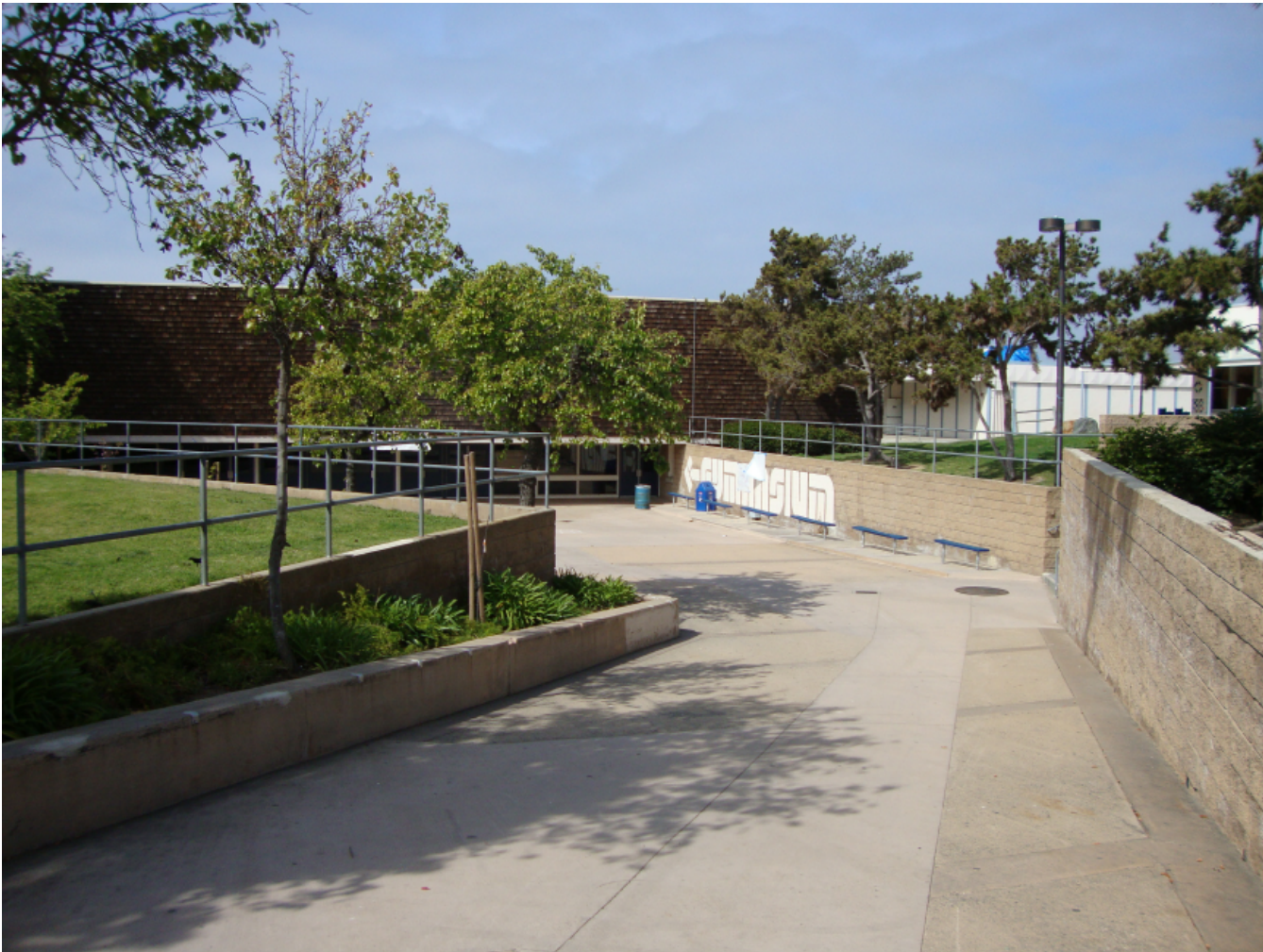
Walkway Leading to Gymnasium East Entrance
