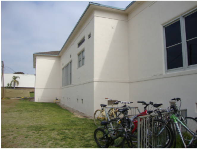
North Elevation of Administration Building B
