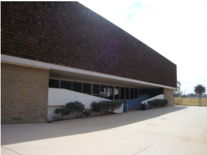
Gymnasium's West Elevation
